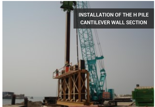
LIFTING PILES INTO PLACE FOR INSTALLATION TO BEGIN
