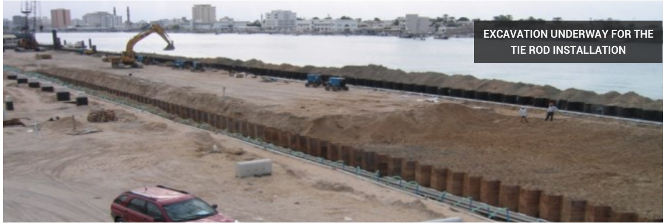
ANCHOR WALL SHEET PILES INSTALLED
