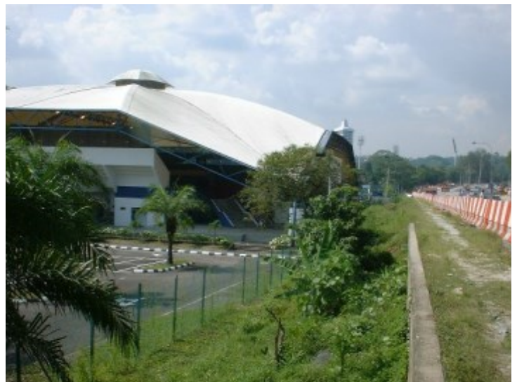
Wall 4 before construction.
