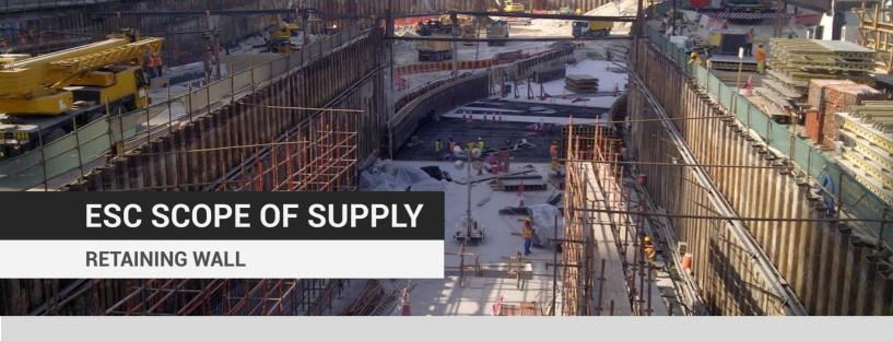
The total length of the temporary sheet pile retaining wall was 790m. Sheet piles of different configuration and length were used to suit the site conditions and the design requirements. The type of sheet piles installed included CR13-575, CR13-600, NSPIIIW and FSPIV with lengths varying between 9.5m and 15m, which correspond to a total tonnage of approximately 1,400T (1,463 nos).
