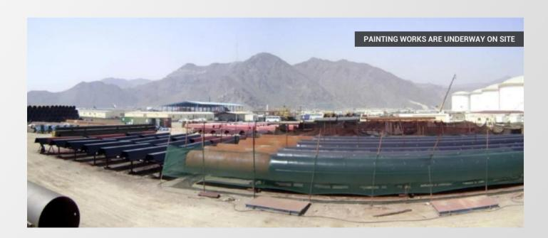
The specified coating for the sheet piles is for shot blasting to SA2.5 followed by 2 layers of 250 micron Jotamastic 87. The coating was applied to the top 22.3m of the front of the ESC Tubular Piles and the back 4m. The ESC Sheet Piles had the full 22m length both sides with paint applied. The ESC Anchor Piles had no coating.
