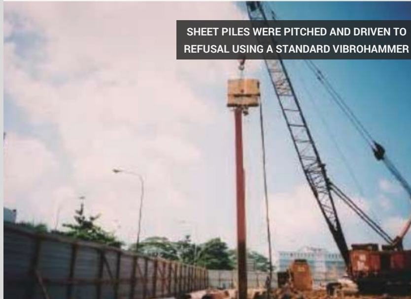
AFTER INITIAL INSTALLATION WITH THE VIBROHAMMER A
