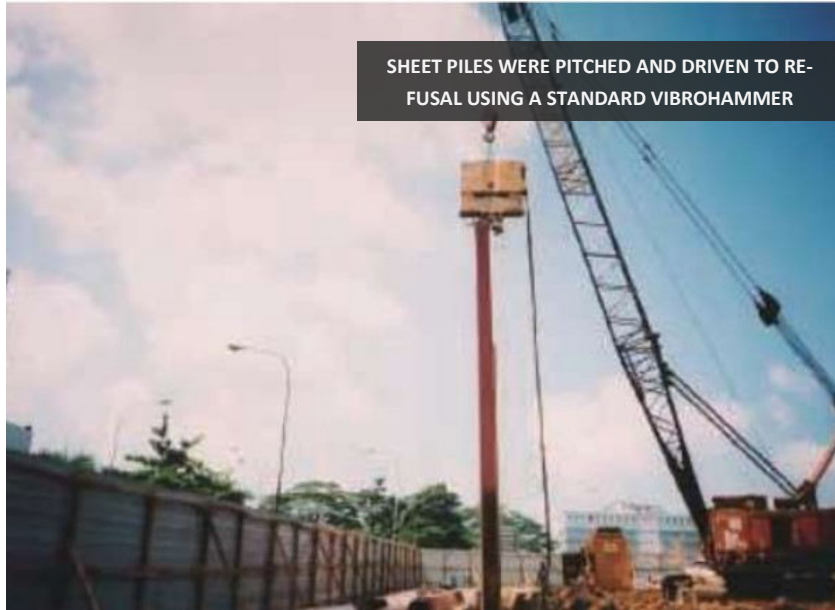
AFTER INITIAL INSTALLATION WITH THE VIBROHAMMER A HYDRAULIC HAMMER WAS EMPLOYED TO DRIVE TO FINAL DEPTH
