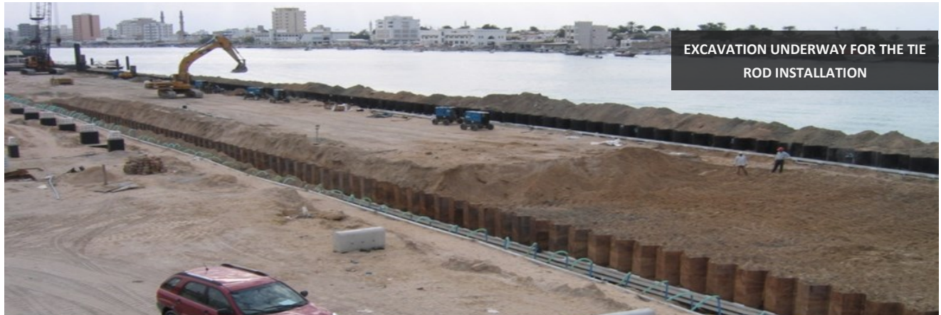
ANCHOR WALL SHEET PILES INSTALLED
