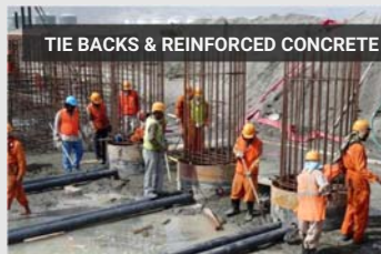
KING PIPE PILES LOADED
