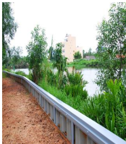
SHEET PILING WITH 2 LEVELS OF ANCHORING
