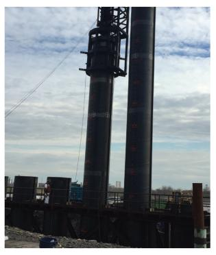
is in the ratio 1:1 to 1:2 with the weight of the pile plus driving cap. A heavy hammer with short drop is always preferable to minimise pile head damage and noise level emissions.
