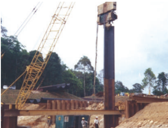
DRIVING USING ESC GUIDE
