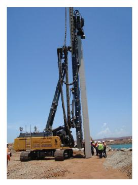
pile. The required driving force is therefore a function of the undrained shear strength of the soil and the surface area of the embedded pile.
