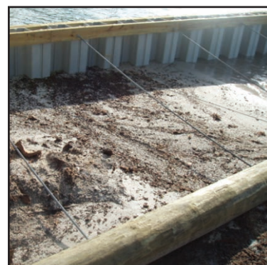
SHEET PILE WALL WITH TIEBACKS
