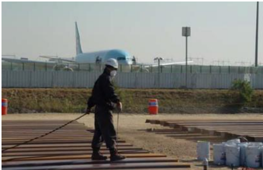
① Sheet piles have to be arranged level.
