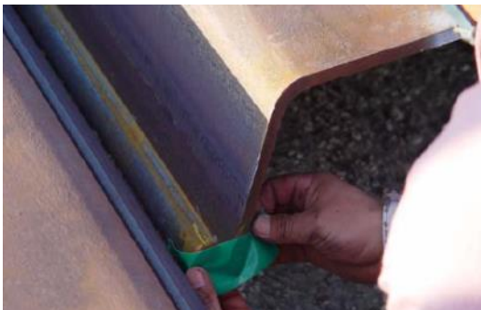
③ Attach small tape to the both sides to prevent the DPS-500 rolls down from interlock .
