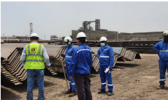
QUAY WALL PROJECT, TAIWAN
