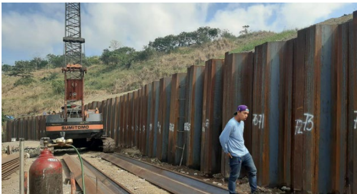
SLOPE PROTECTION, PHILIPPINES
