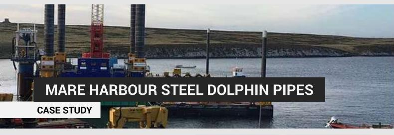
ESC Steel Structures fabricated and supplied 13 steel mono piles to Edgen Murray Europe. The project was part of the Mare Harbour base improvements in the Falkland Islands. Each steel dolphin pile included fender mounting brackets and stiffeners, bollard supporting plates and topside deck plates.
