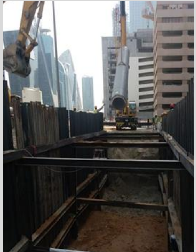
ESC TRENCH SHEETS INSTALLED AMIDST BUSY STREET IN
