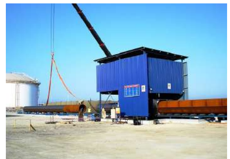
BLASTING OF PAIRED SHEET PILE
