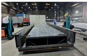
STEEL MOULD FABRICATION
