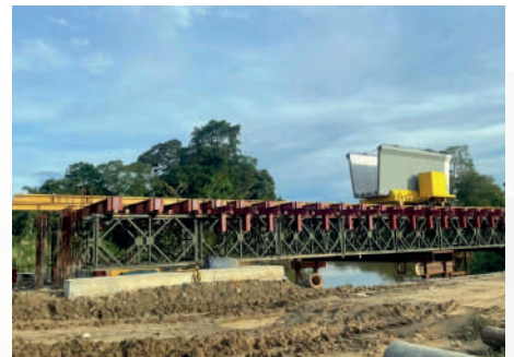
MODULAR STEEL BRIDGE, PNG
