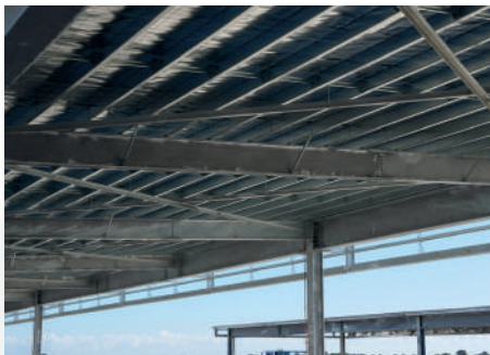
AIRCRAFT HANGAR, AUSTRALIA
