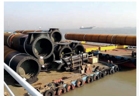
DOLPHIN PIPES, FALKLANDS
