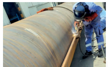
STEEL PIPES INTERLOCK FABRICATION
