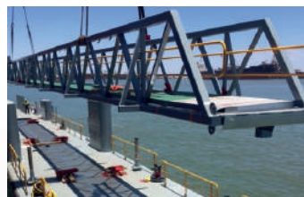
GANGWAYS AND PLATFORMS
