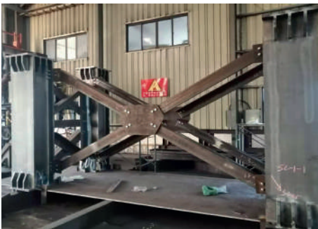
HEAVY BOX COLUMN FOR AUXILIARY STRUCTURE, PHILIPPINES
