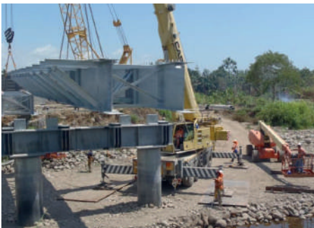
BRIDGE GIRDER, PNG
