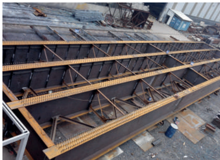
NEW BRITAIN BRIDGE PROJECT, PNG
