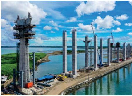
BRIDGE STRUCTURAL STEEL SPUDS, PHILIPPINES
