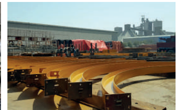
AMPLE MATERIAL STORAGE CAPACITY
