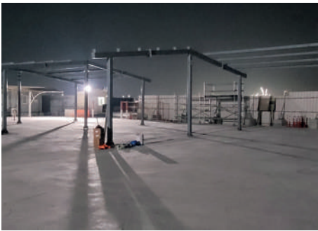
CAR SHED, UAE
