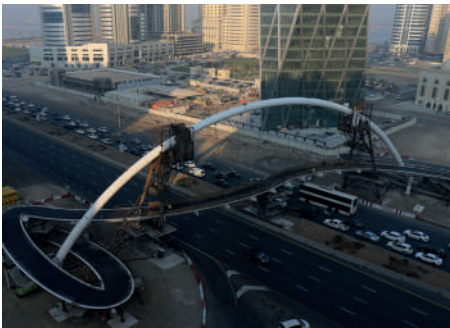
AL ITTIHAD FOOTBRIDGE ARCH, UAE
