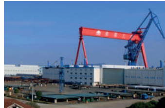
OUTSIDE FABRICATION & STORAGE
