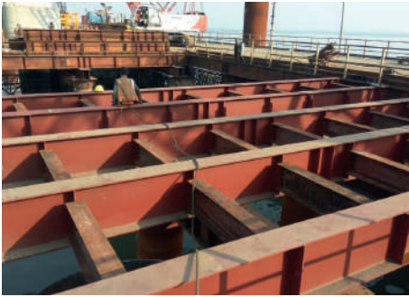
MUMBAI TRANS HARBOUR LINK, INDIA
